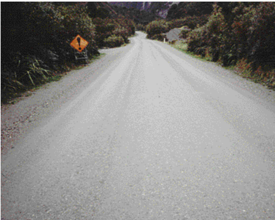
This road in New Zealand performs remarkably well because of good crown and good gravel quality in a region that receives nearly 150 inches of moisture a year! (Courtesy of Ken Skorseth, SD LTAP)
