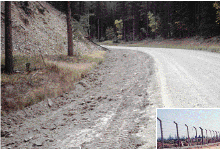
A nicely reshaped ditch that meets the shoulder line of the road and allows good drainage.
